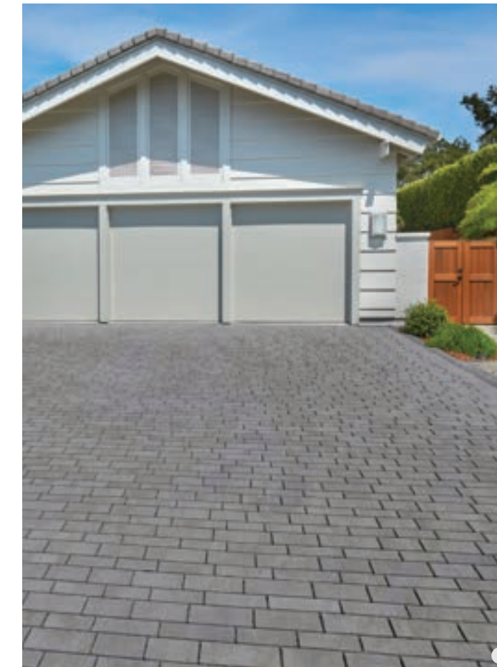
1. Dark Gray-Pewter-Charcoal Permeable Aqualina installed in a random runner pattern. 2. Permeable Aqualina pavers are installed over an open-graded base and with rock chips in the paver joints instead of sand to allow water to flow into the base underneath the pavers. 3. Dark Gray-Pewter-Charcoal Permeable Aqualina installed in a random runner pattern.
