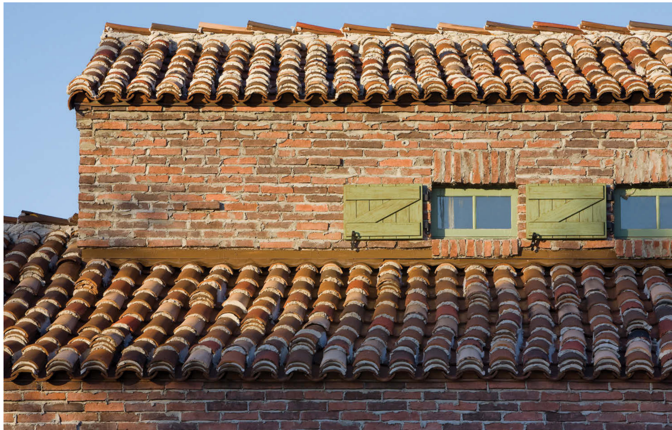
Bracciano RomaBrick (pg. 78) with an overgrout technique.
