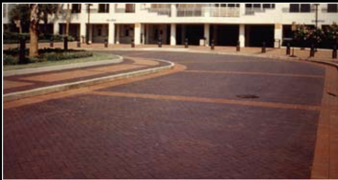
Marion Street Transit Tampa Bay, Florida 2-1/4 x 4 x 8 Pavers Medium Ironspot #46 Medium Ironspot #77
