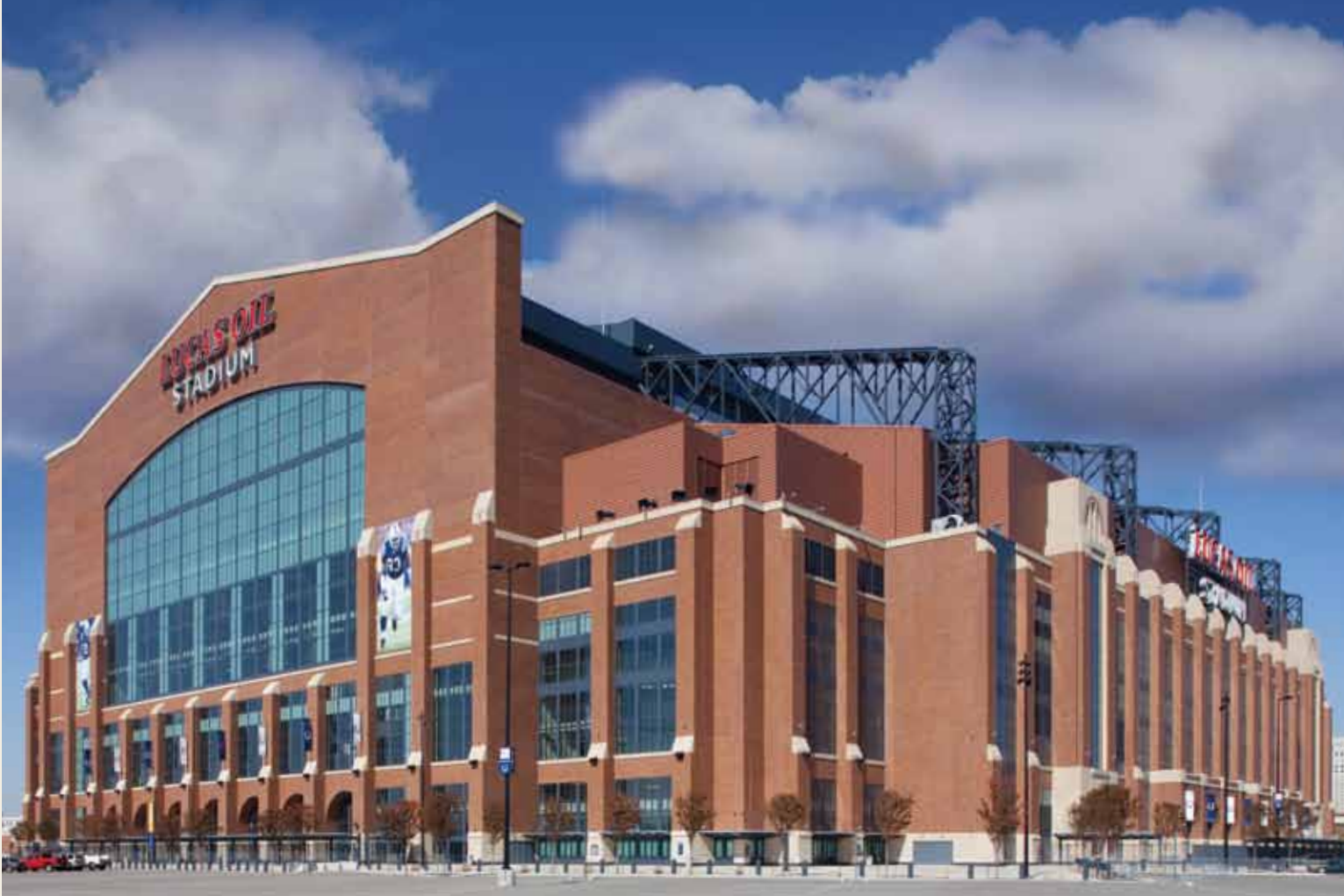
Lucas Oil Stadium – Indianapolis, Indiana Medium Ironspot #77 (Field), Manganese Ironspot (Accent) Thin Brick Precast; 1/2" x 3-5/8" x 7-5/8" (Utility) Velour Texture
