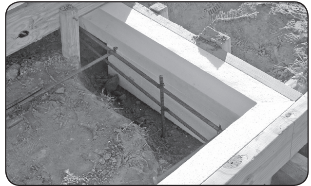
Use spray adhesive/ nails to attach.
